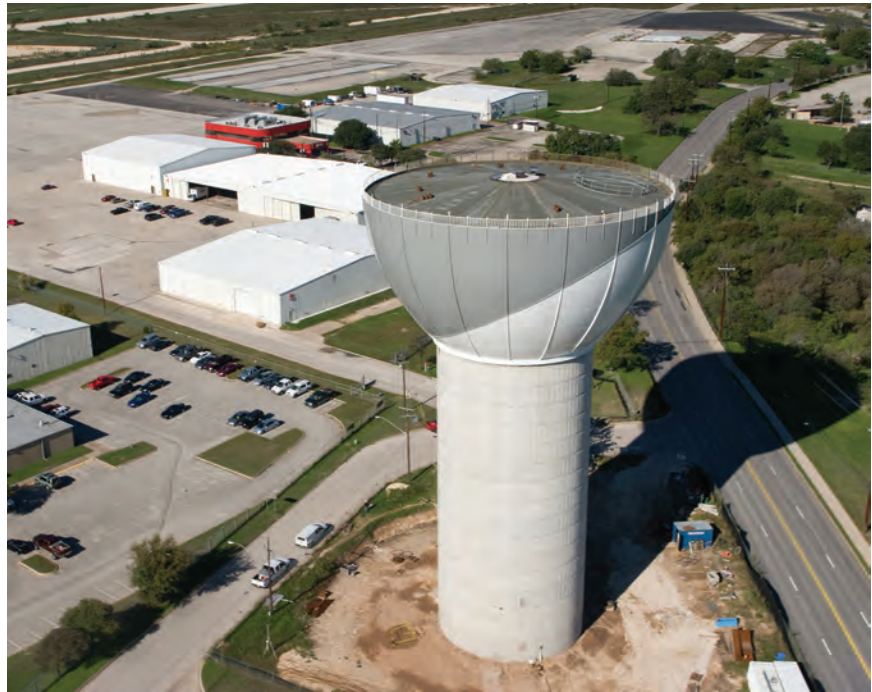
The 170-ft-tall tank is positioned on a compact site bound by existing roads and structures.
