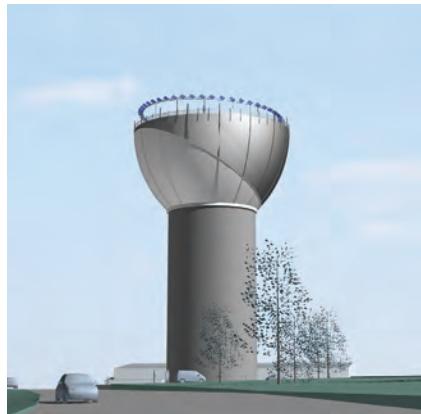
The rooftop accent ring will support 48 PV panels for solar power generation.
